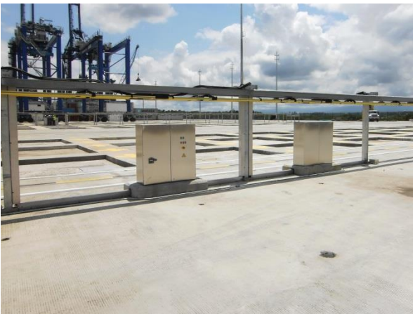
Caption: Pillar Boxes and E-RTG Drive-in L systems in back-to-back arrangement
